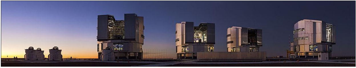
Figure 10: ESO's Very Large Telescope at Cerro Paranal, showing the buildings that house the four 8.2-m telescopes, which can be used individually or as an interferometer ( en.wikipedia.org ).
