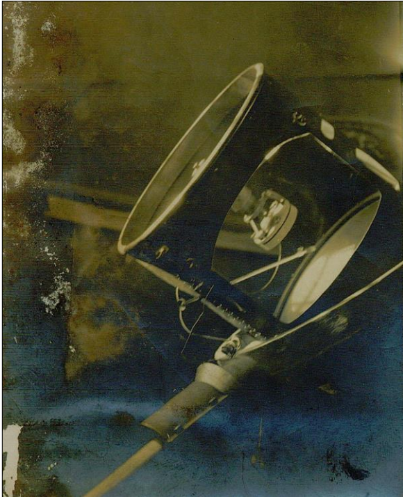
Figure 1: Photograph of the 30-inch as solar furnace in the laboratory of Elmer Gates circa 1906 (image used with the permission of Elmer Gates.com.).
