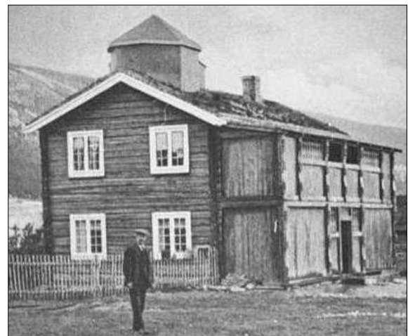
Figure 4: The house at Brennøygarden with the roof-top observatory. Sigurd Enebo is posing in the foreground (courtesy: Urd 27 March 1915; photographer: H.H. Lie).
